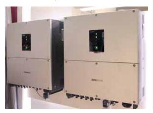
Problem: 1,500V solar systems are expected to dramatically reduce system costs and improve power generation efficiency. The solar industry has long demanded a 1,500V string inverter to reduce the levelised cost of electricity for commercial- and utility-scale PV power plants.
