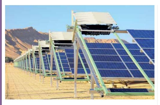
ing a specially designed soft brush that minimises the abrasion visited on the module. Another advantage of automated cleaning he says is its responsiveness to sudden soiling events such as sand or dust storms. Ecoppia's solution is operated via the cloud, with sensors at the site keeping a constant check on particulate levels, and issuing instructions to clean if they pass a certain threshold. That means cleaning can be underway in next to no time.
