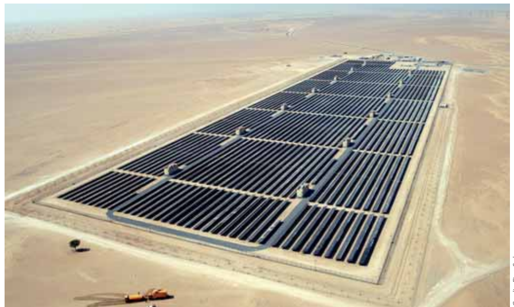
Credit: First Solar
