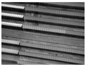
Figure 4. Disconnected string detected with aIRT on a singleaxis tracking, utility-scale PV power plant
