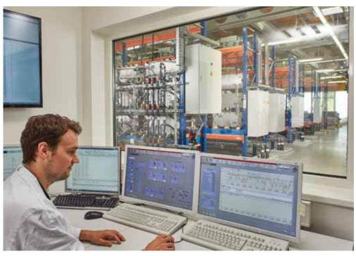
Figure 6. Control room of a 2 MW/20 MWh vanadium redox flow battery at Fraunofer ICT
