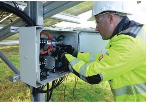
Commissioning is vital in ensuring a PV power plant operates as expected over its lifetime
