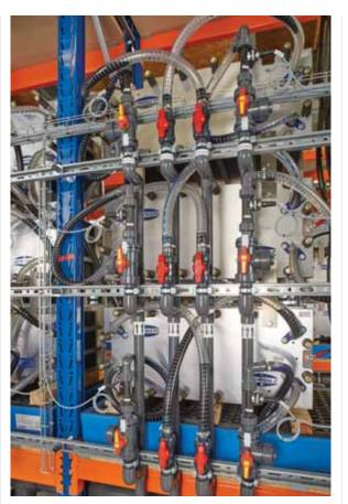
Figure 8. Piping and stacks of a 2 MW/20 MWh vanadium redox flow battery at Fraunhofer ICT
