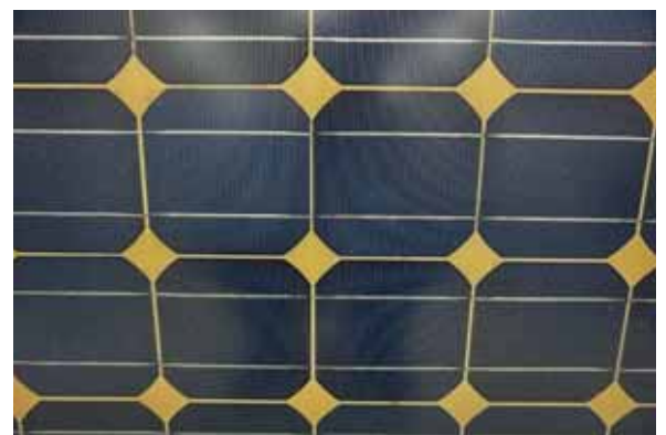
Figure 4. Nine-year-old field module in Tibet with a polyester backsheet: the backsheet inner layer is yellowing and the outer layer is cracking and peeling off
