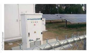
A DC-coupled battery at Duke **Energy's Mount** Holly test site. Expectations are high that DC coupling will help drive down solarplus-storage costs
