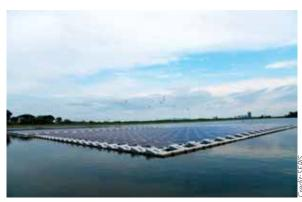
Figure 1. Ciel et Terre's floating solar mount is an example of the pure-float design
