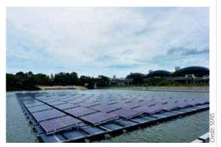
Figure 2. Takiron Engineering is one company producing the pontoon + metal frame variant of the floating solar mounting structure
