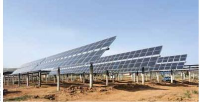
The addition of larger, heavier modules to existing tracker designs will require more thought when it comes to wind.
