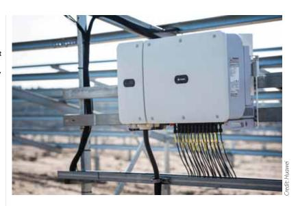
need to be connected to the inverter, but this means the other inputs and available MPPTs that are available are being wasted. The problem is exaggerated even more when using strings of longer than 30. Inverter manufacturers have a tricky job to guess which large-format design is going to win out, and to create products that are better tuned to the new generation of modules.
