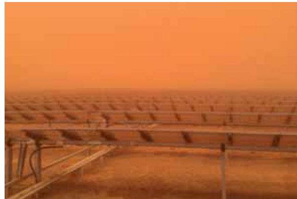
Figure 2. A solar PV plant in the midst of a severe sandstorm in Jordan
