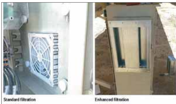
Figure 7. Standard versus enhanced array box filtration
