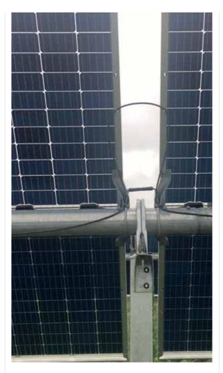
current industry 32A in-line fuse rating, the BGF factor assumption can result in the purchase and installation of up to two times the number of wire harnesses as compared with an equivalent monofacial project.
