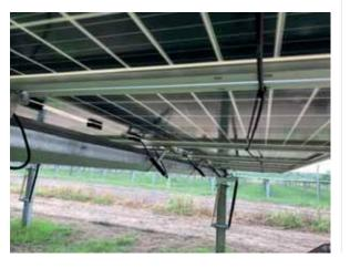
Figure 1. Wiring considerations for bifacial modules: to prevent shading of the rear-side of the module how the DC wire harnesses will travel down the racking structure without shading the rear side of the modules must be considered during the design and procurement stages of the project. Different modules paired with different racking structures require custom approaches
