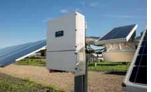
the entire solar power array to a safe 60 degree stow angle. This action will have the benefit of up to tripling the hail resistance module toughness and dramatically reducing damage potential, according to independent tests carried out by RETC (Renewable Energy Test Center). In the case of snow shed, an authorised operator can pre-schedule two snow shed operations in a single day, which increases production by reducing snow cover on solar panels.
