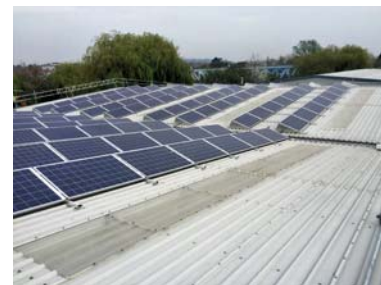
Upstanding South Facing system on East/West pitches
