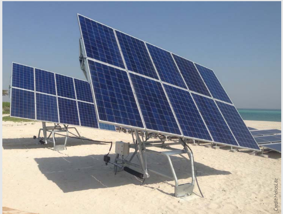
HeliosLite's 1.5-axis tracker is claimed to be suited to niche markets where mainstream trackers are less well adapted
