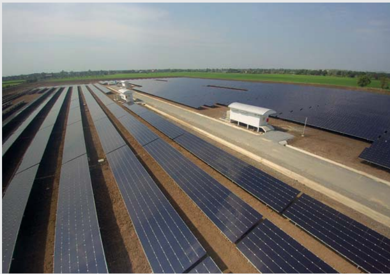
Credit: First Solar
